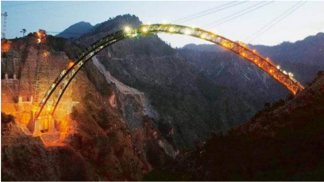
Chenab Bridge under construction at night
