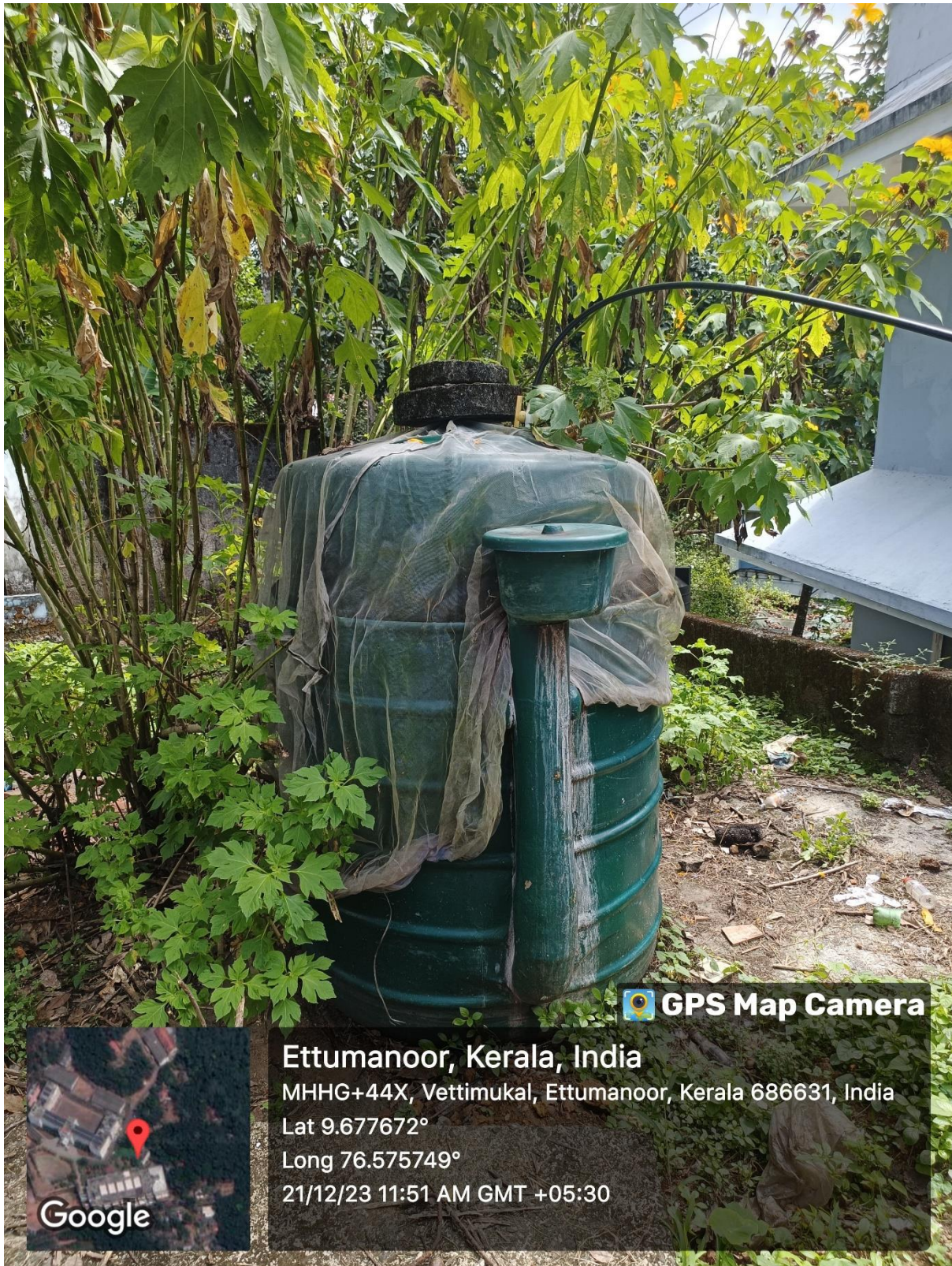
Fig 4, Biogas Plant
